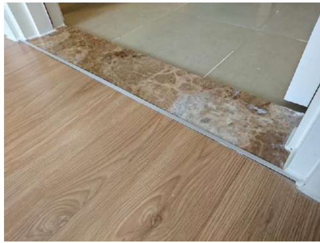
■ CONDOMINIUM (HO CHI MINH/VIETNAM)
