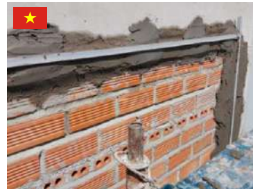
Formwork Joint Bar
