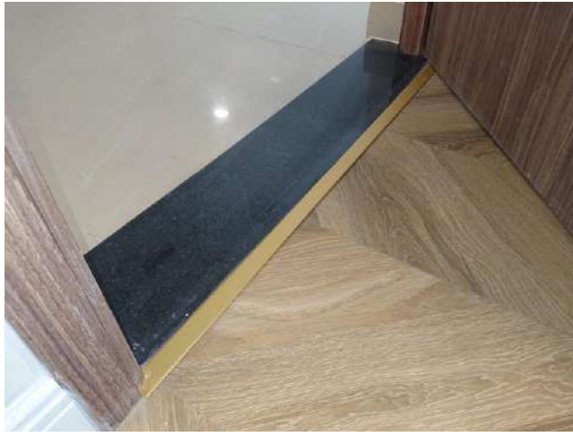
■ CONDOMINIUM (HO CHI MINH/VIETNAM)
